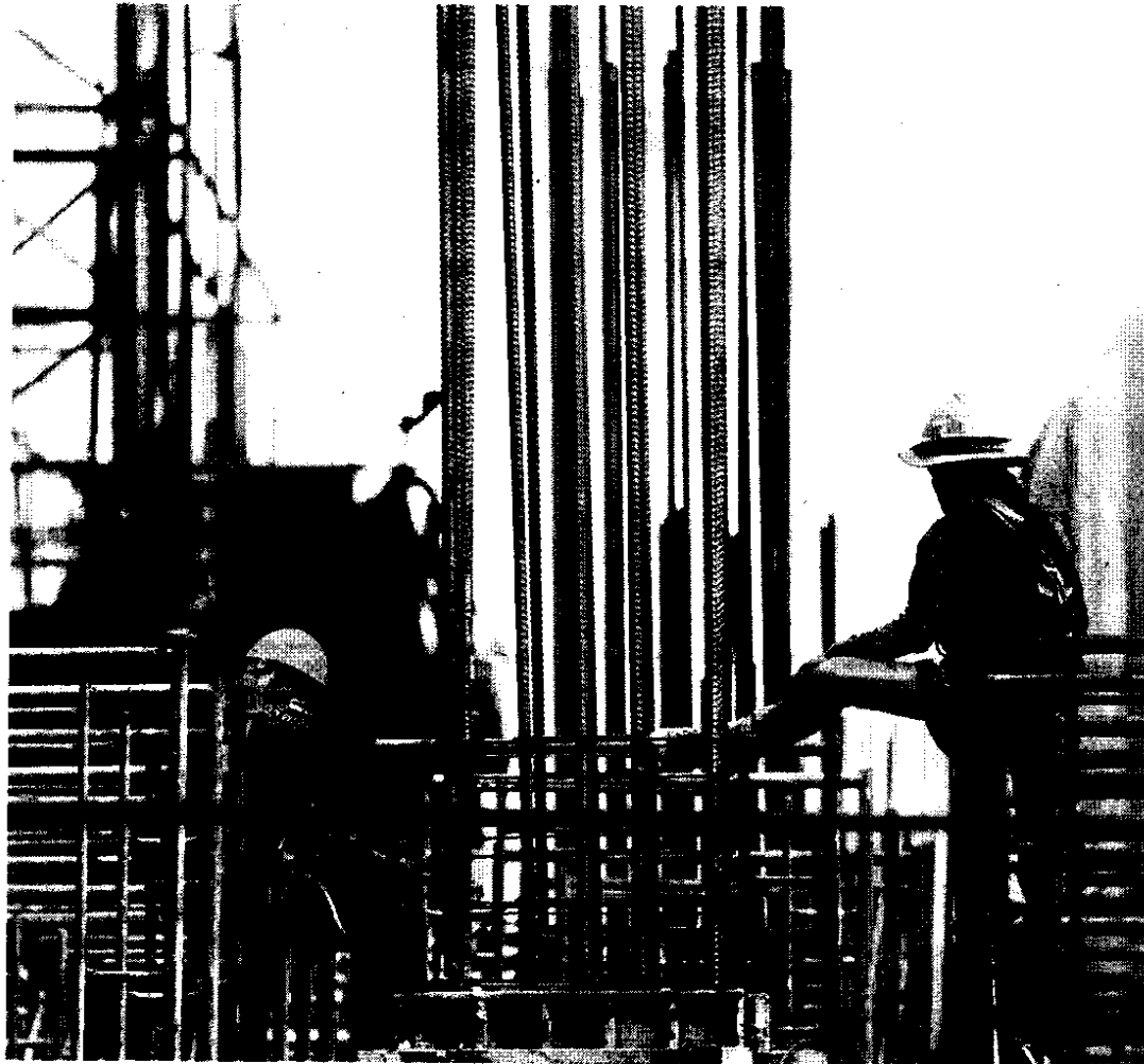
A condominium construction site in Bangkok. Private investment is expected to be a key economic driver next year. SEKSAN ROJJANAMETAKUN
