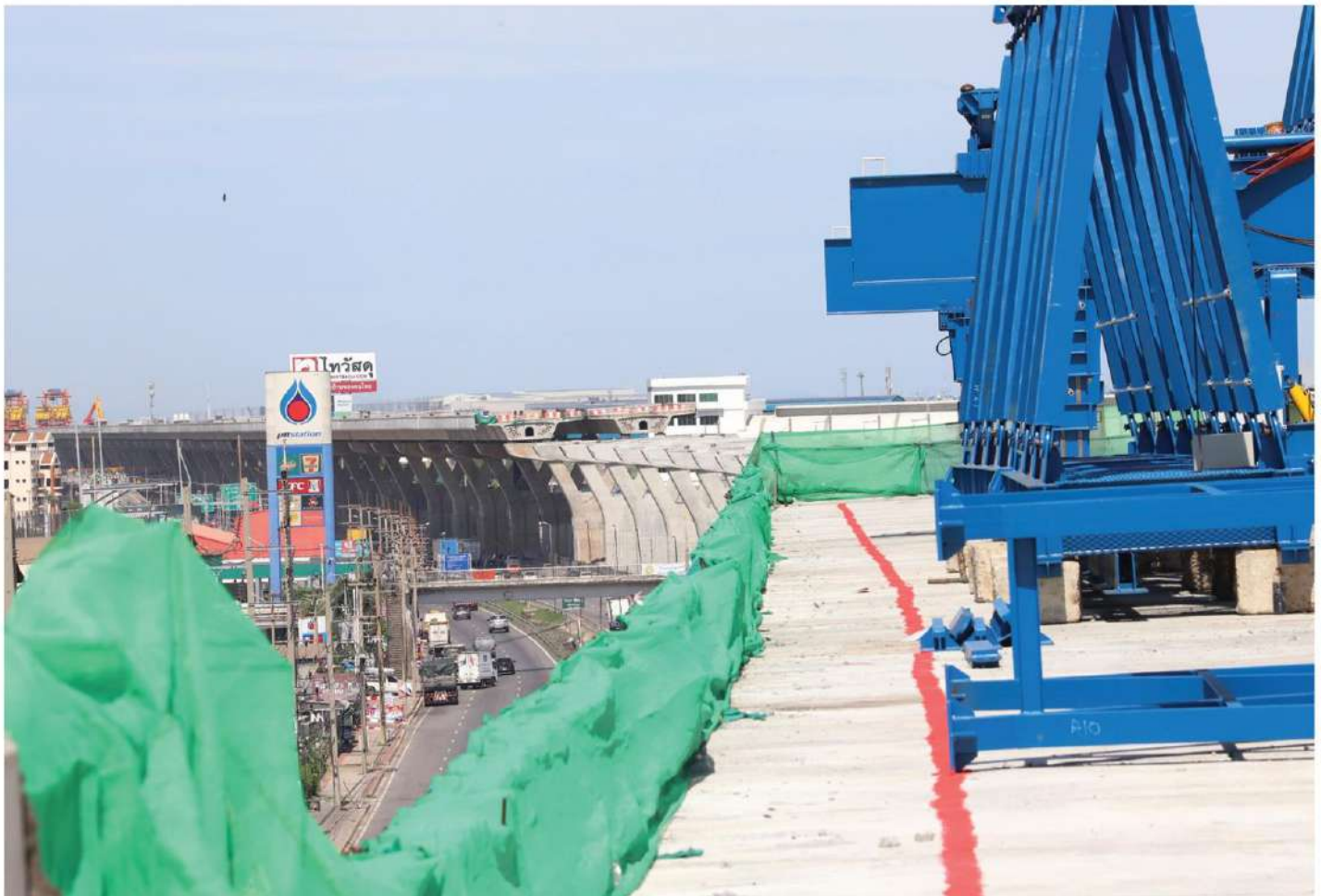
Construction work continues on an elevated section along Rama II Road. Mr Ekniti says state spending is the only engine capable of pulling the Thai economy out of its current slump. Photo: Apichart Jinakul
