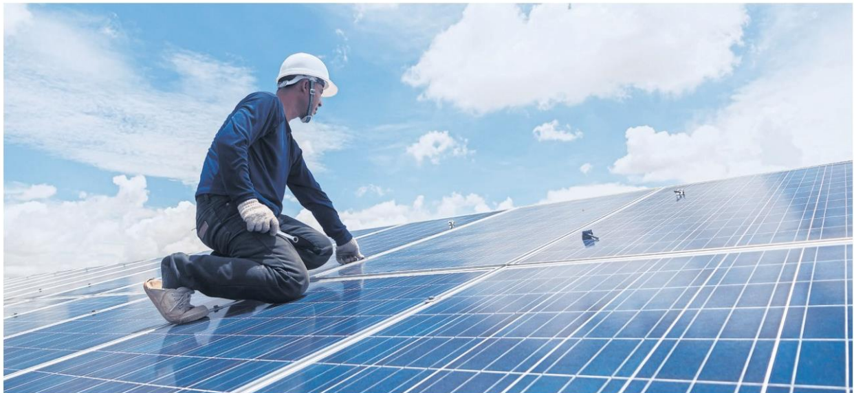
An engineer replaces a solar panel on the roof of a solar power plant. The community solar cell project is one of three projects the government aims to push forward to completion by the end of this year.
