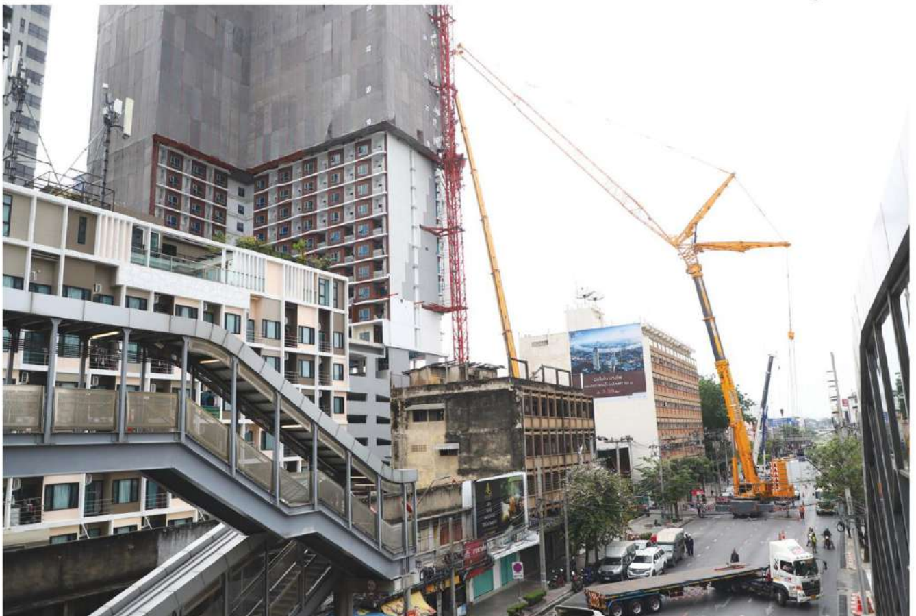
Workers dismantle a damaged crane at Niche Mono condo project in Bang Sue district, which collapsed in the earthquake on Friday. PORNPROM SATRABHAYA
