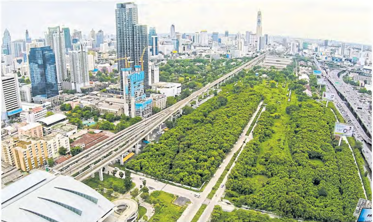
An aerial view of the State Railway of Thailand's Makkasan plot that the Treasury Department leases. KRIT PROMSAKA NA SAKOLNAKORN
