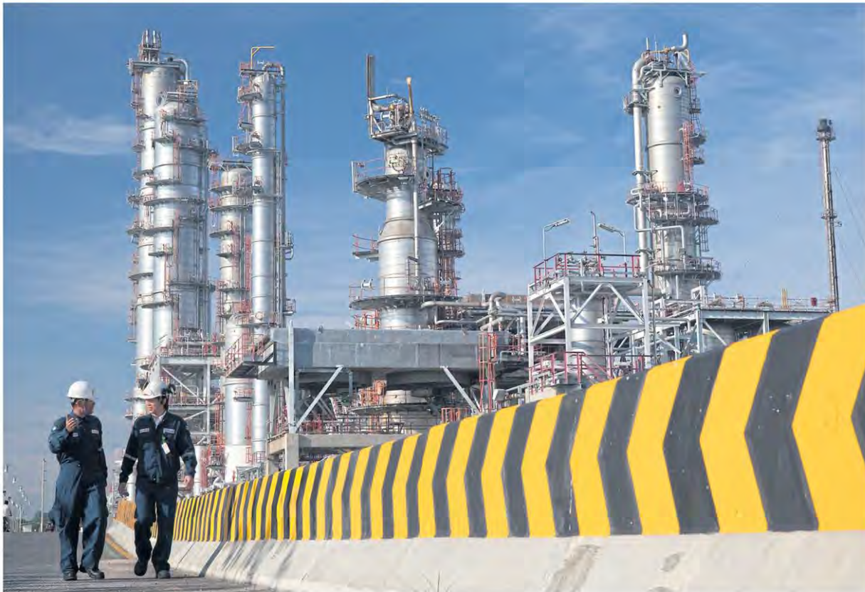
This aromatics plant is part of the Esso refinery complex in Sri Racha. The refinery has a maximum rated capacity of 174,000 barrels per day.
